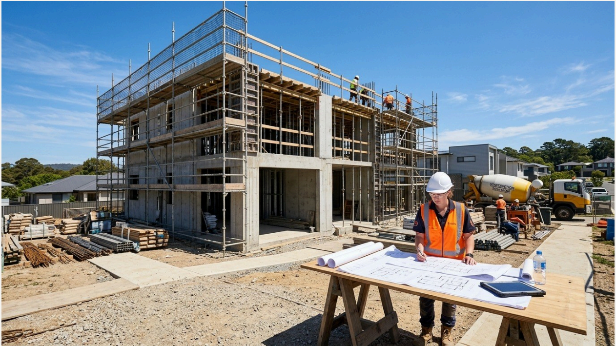
A residential construction site with a site engineer reviewing drawings
